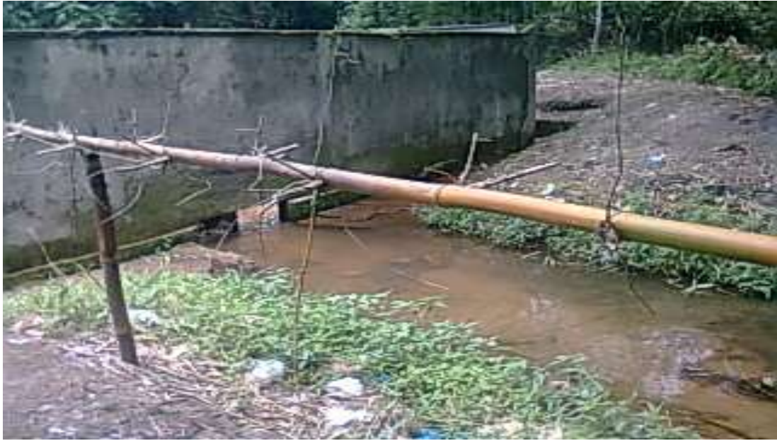
Appendix30: Plate of the Direction of the Out flow Water from the Bathrooms
