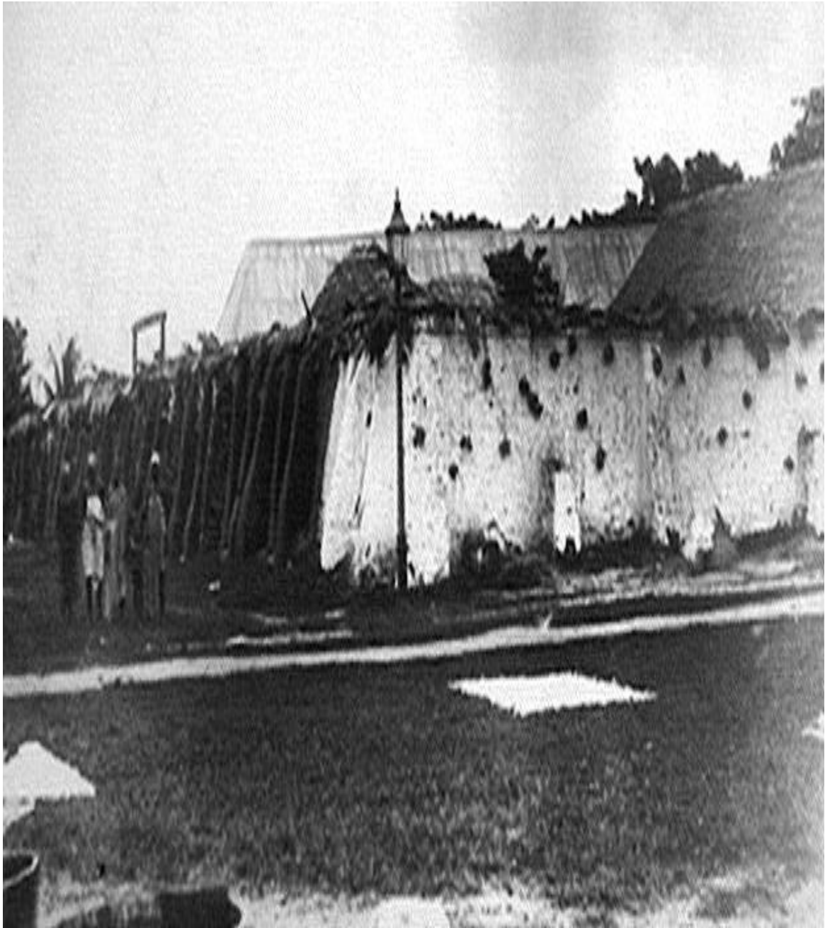
Picture 2.4: Broad Street Prison, Lagos, c.1872
