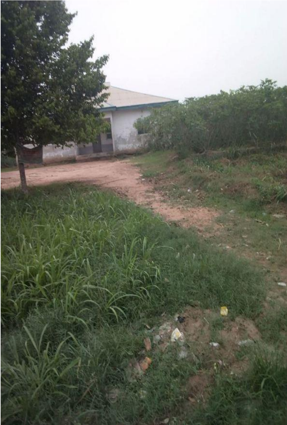
Plate 4.1. The primary health care building at Mbaraikoro village. This replaced the police station that was here in the 1980s after a violent protest caused by an accident that led to the death of a pregnant woman at a police checkpoint.
