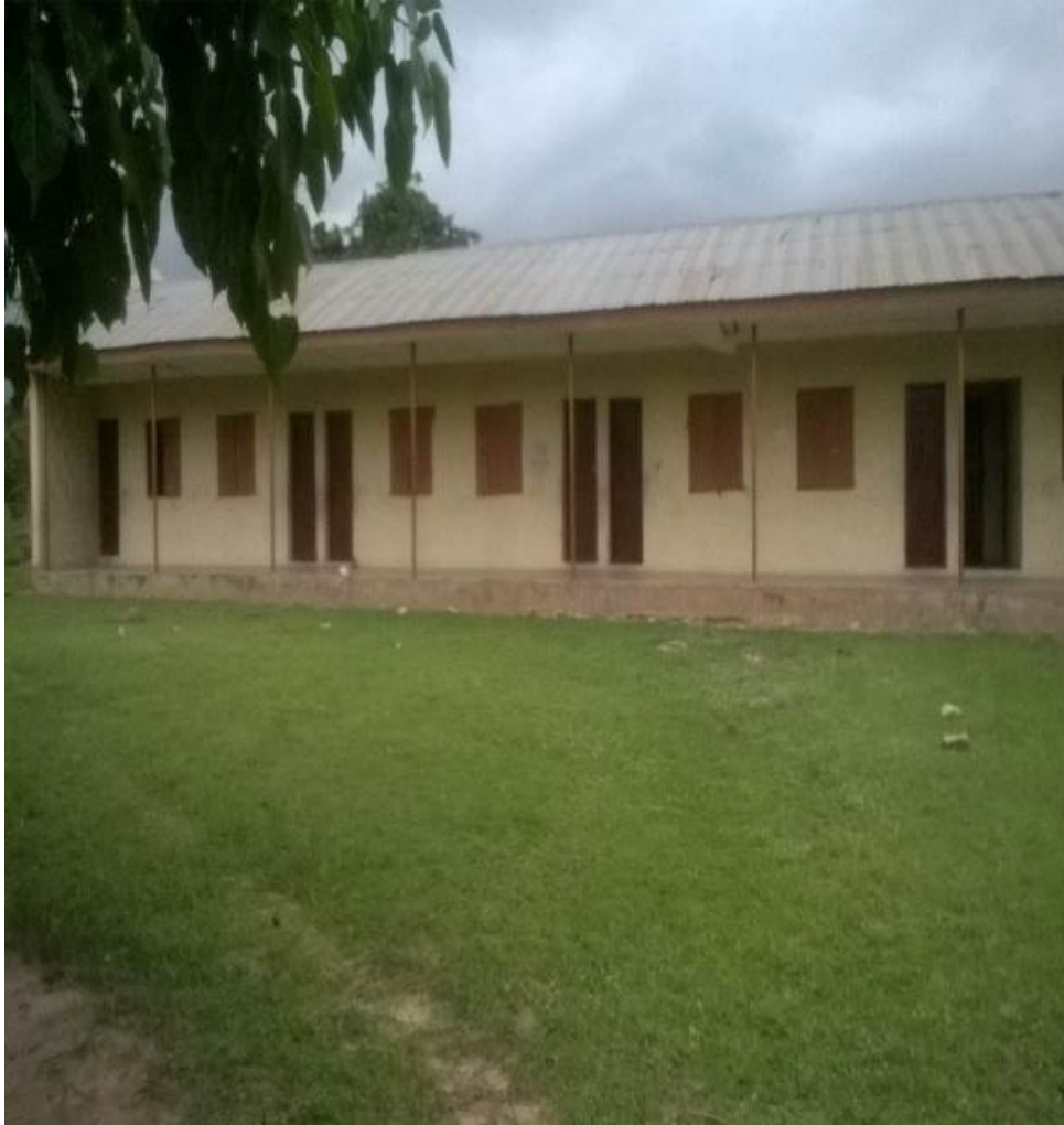
Plate 2: Classroom Buildings of the Nomadic Primary School, Tede (Fieldwork, Tede 2017)
