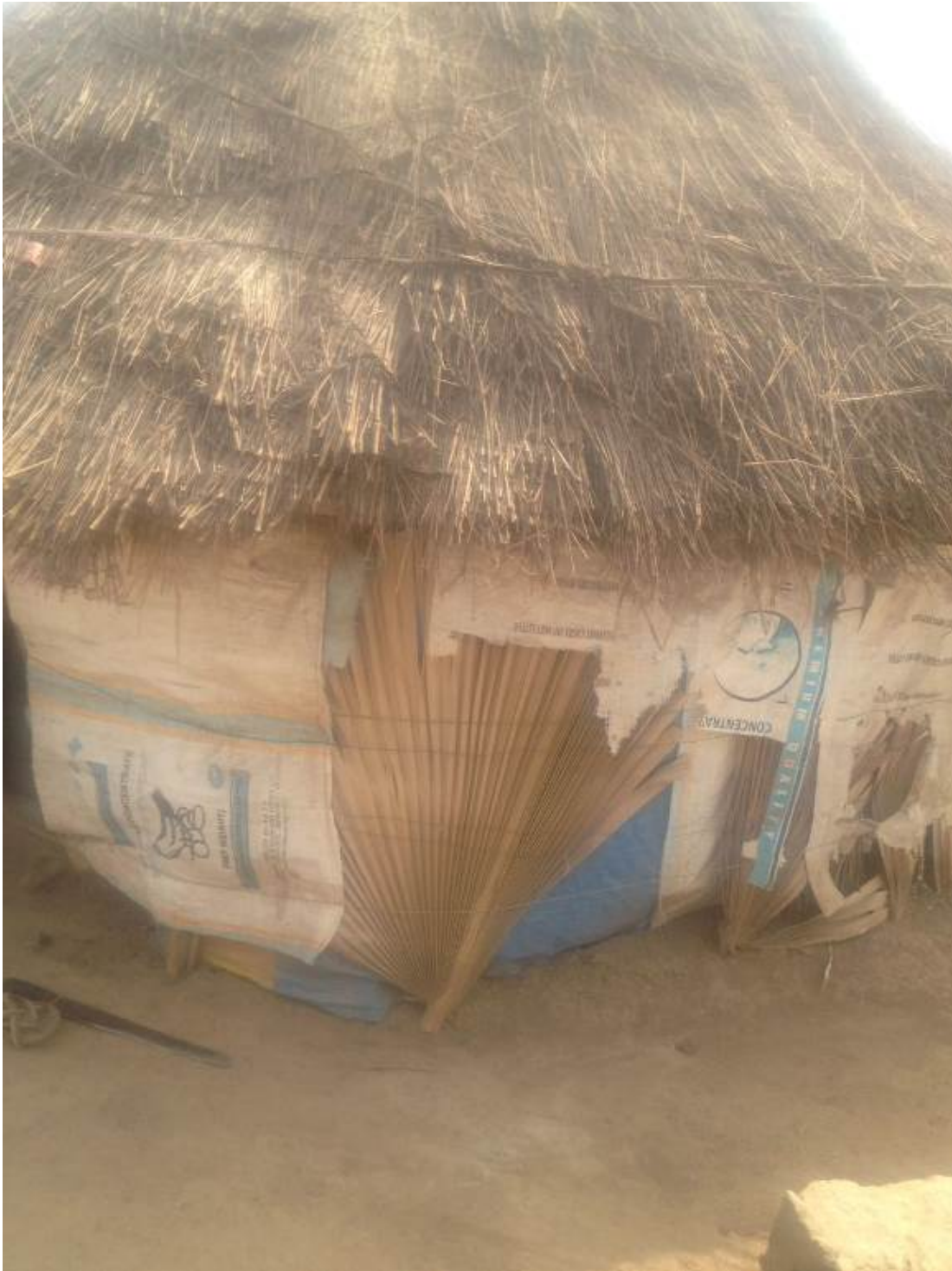
Plate 22: A Fulani Homestead Constructed from Sacks and Other Synthetic Material (Iseyin, Fieldwork, 2017)
