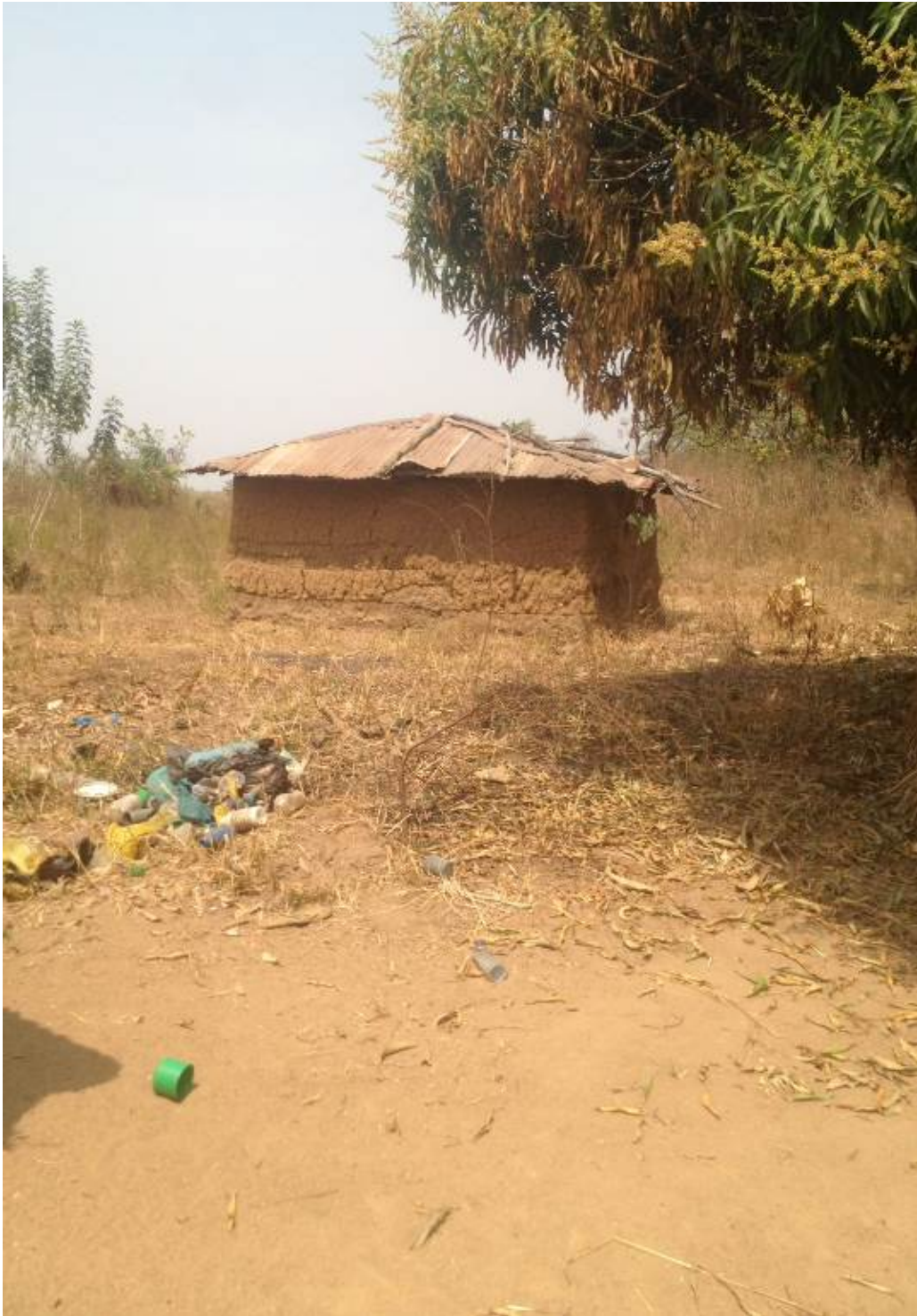
Plate 26: A Fulani Homestead Modern Corrugated Iron Roofing. (Fieldwork, Awe, 2017)
