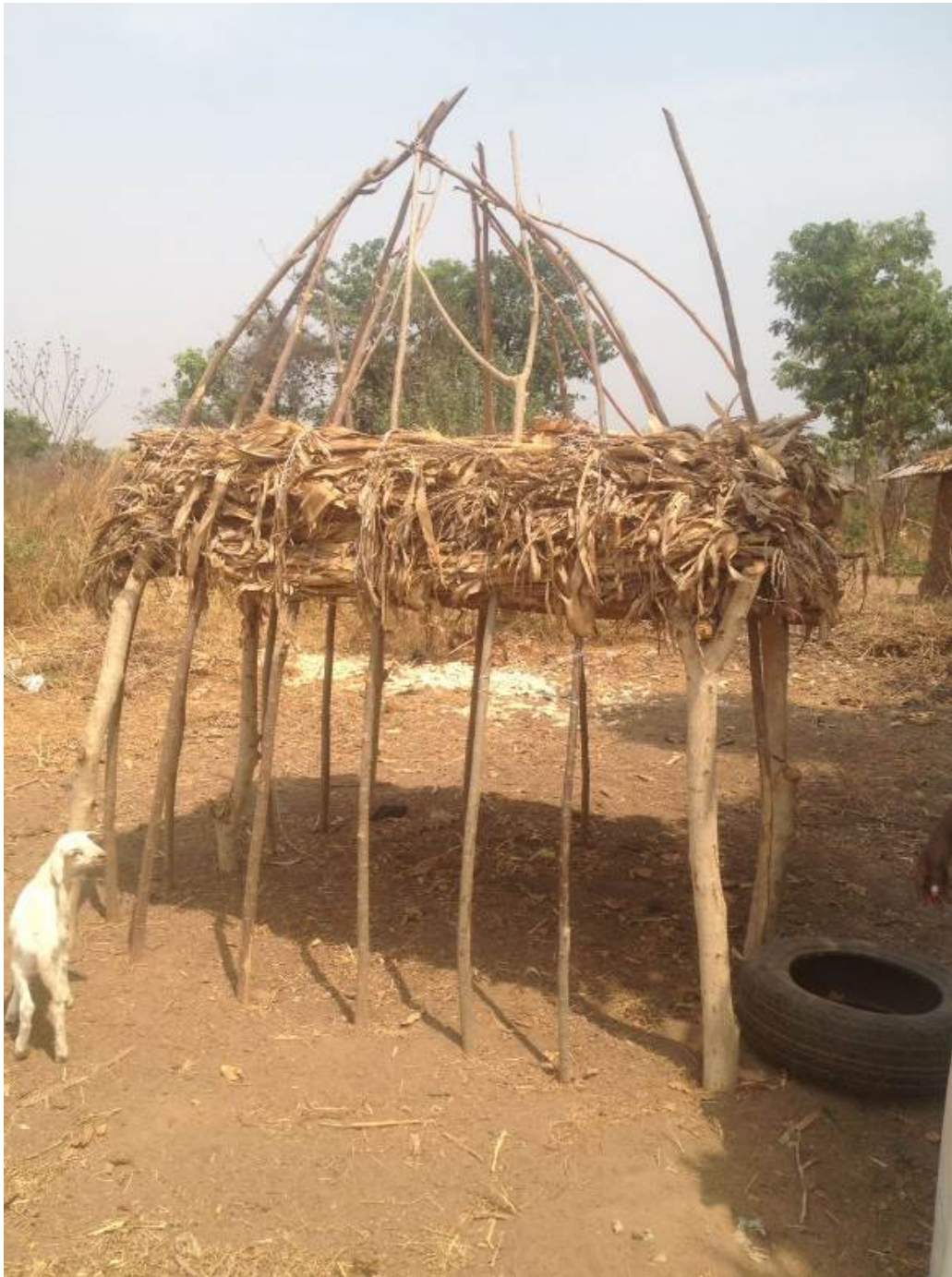
Plate 16: A Granary under Construction. (Fieldwork, 2017)
