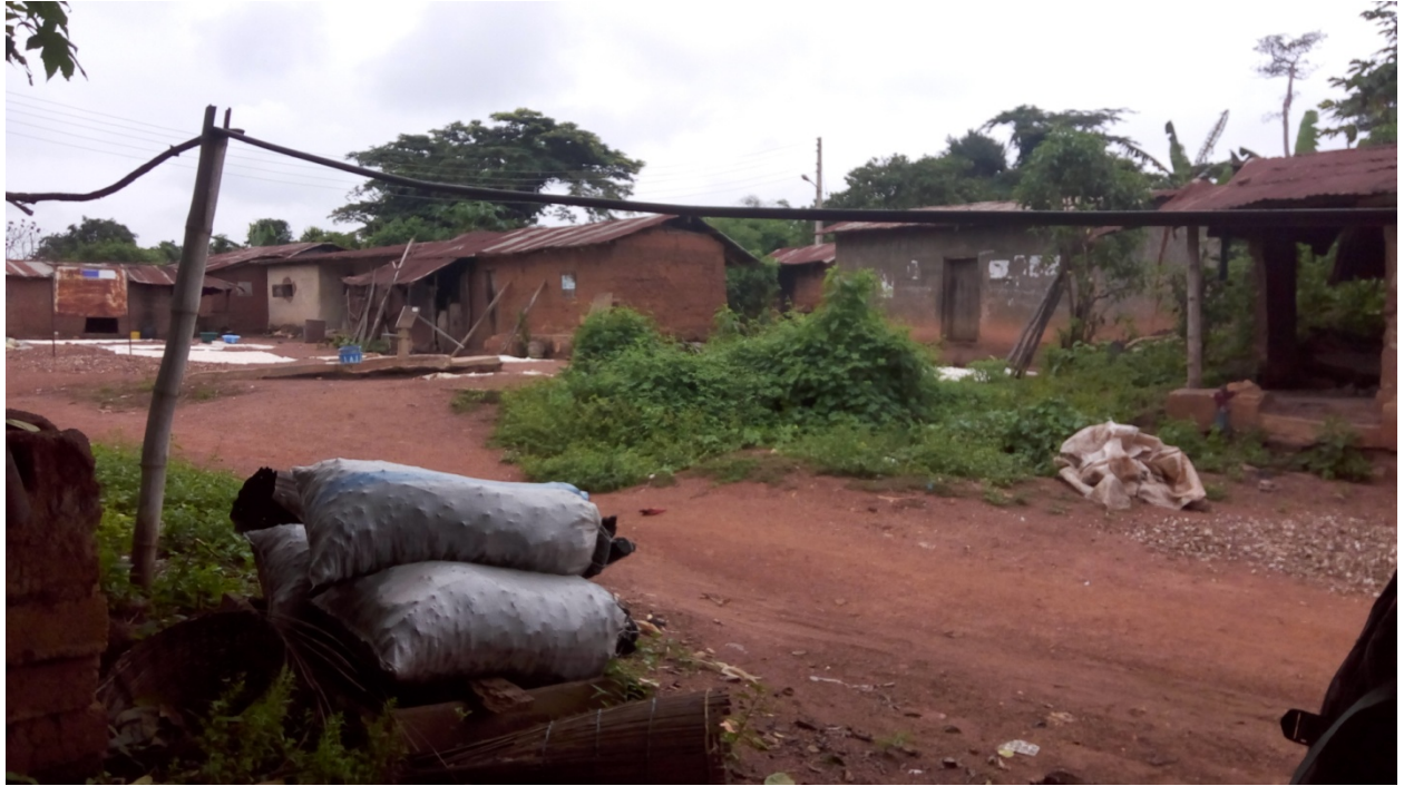
Plate 6: A cross section of the housing type that most rural households secure Source: Field survey, 2017
