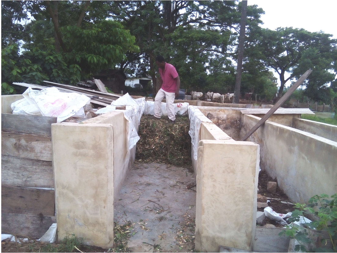
Plate 8: Manual Compaction of silage Materials in the silo
