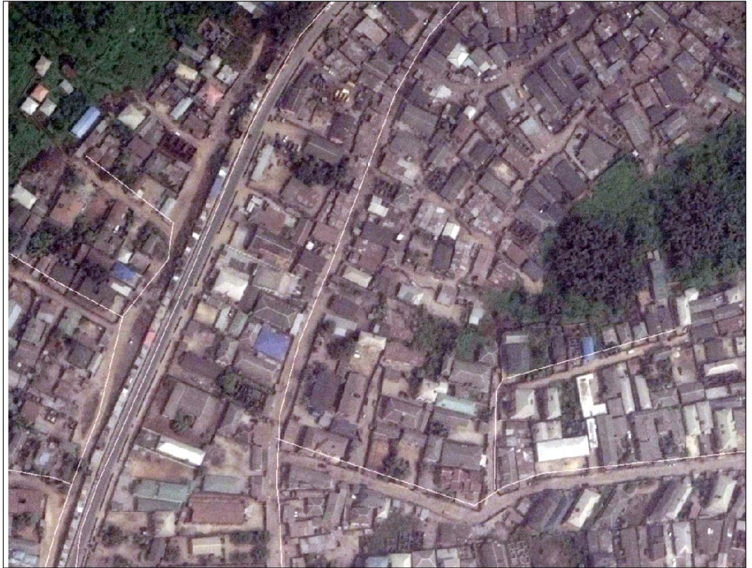
Plate 5.3: Compactly Built but unorganized Section of Isasi in the Western fringe
