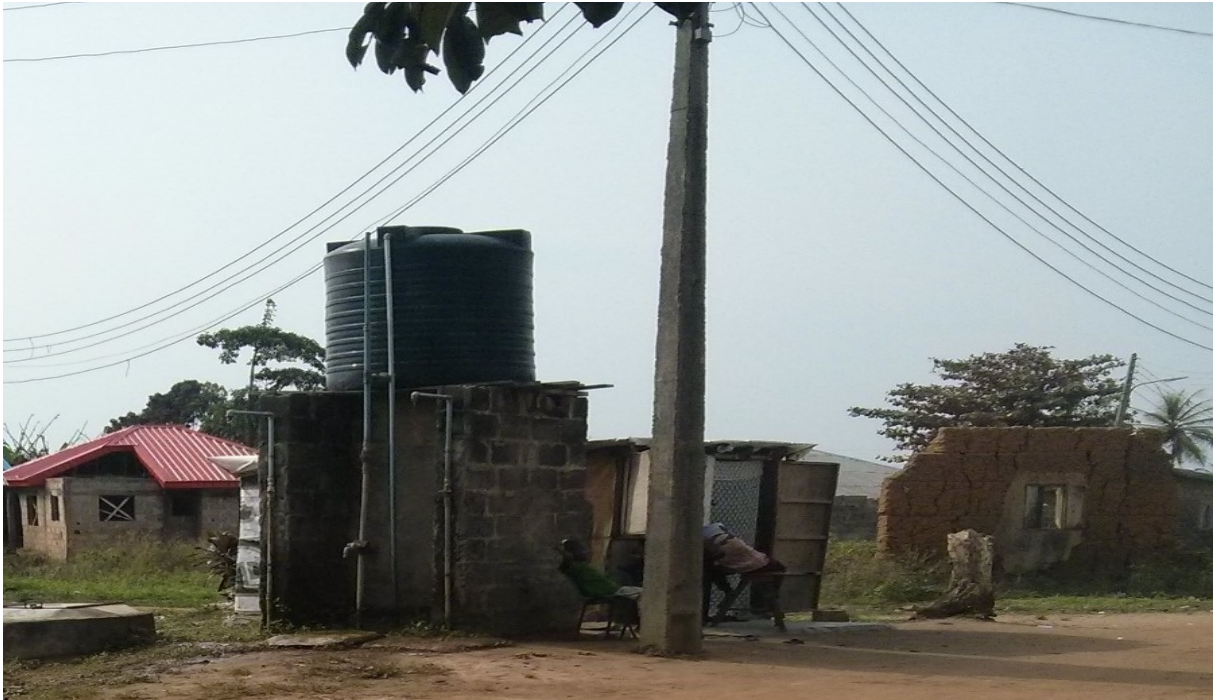
Plate 7.4: Public Borehole at Isefun Community
