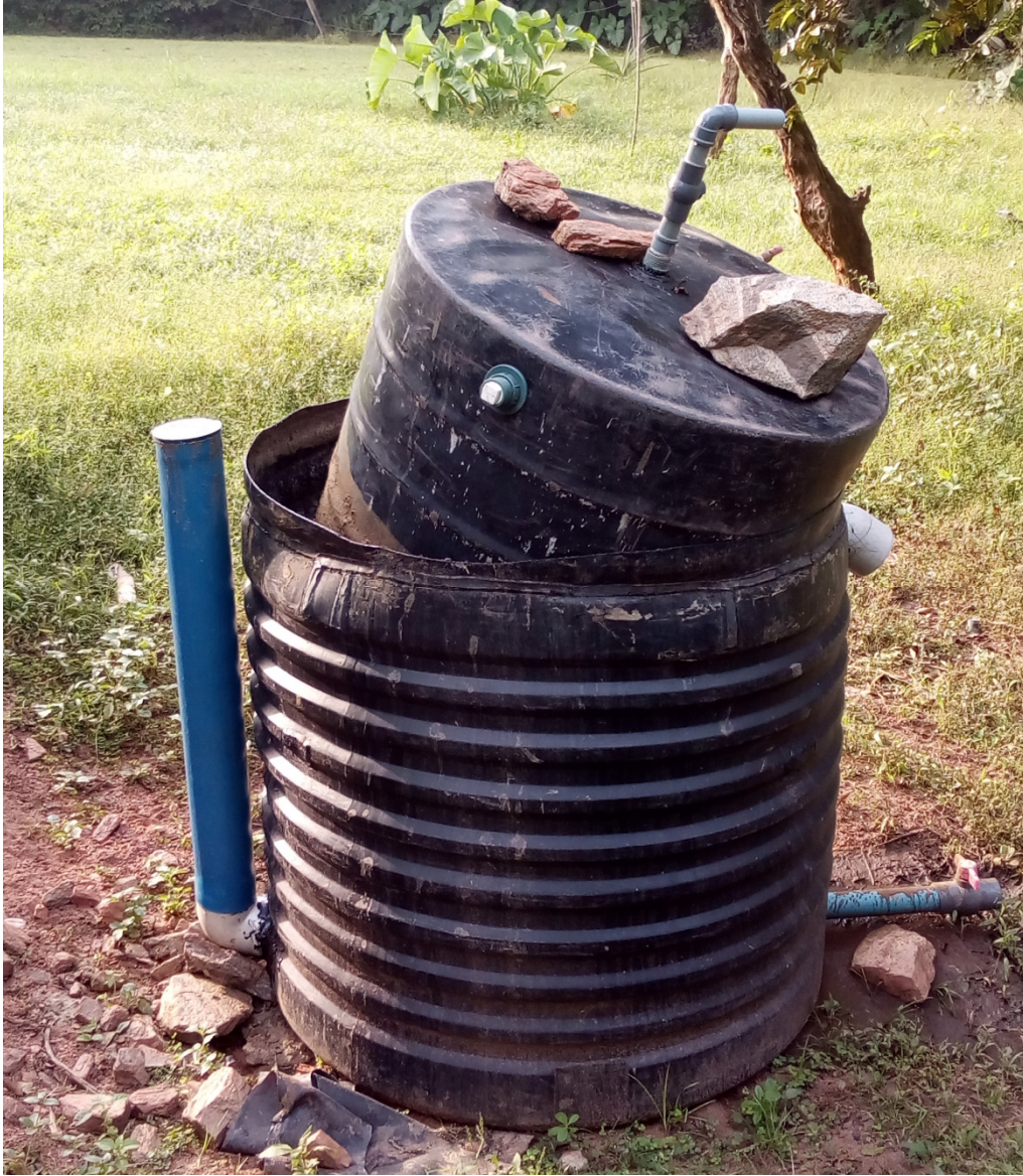
Digester with weight placed on the top to prevent toppling of gas cap during biogas generation
